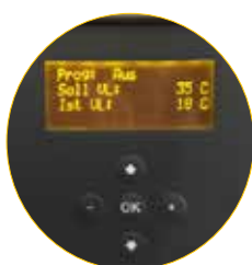
Digital control panel
